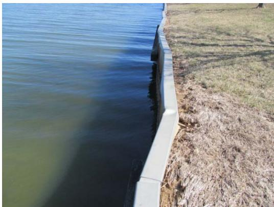
Aluminum bulkhead displaced
