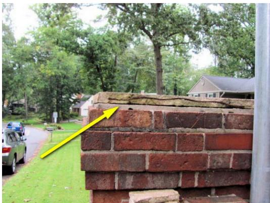
Broken concrete cap
