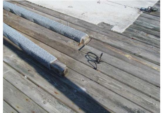
Damaged decking on floating platform
