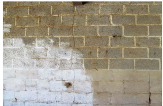
Cracks in CMU wall (minor but need to monitor)
