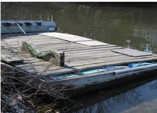
Typical floating platform w/ damaged deck & structure
