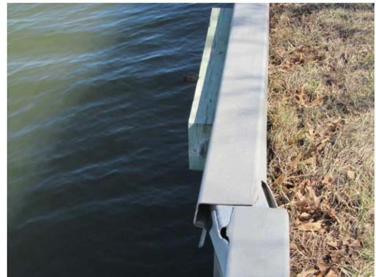
Aluminum bulkhead reinforced with wood rail
