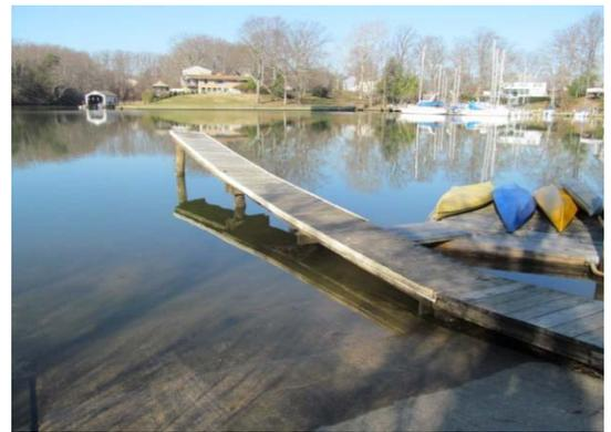
Ramp pier damaged by ice uplift
