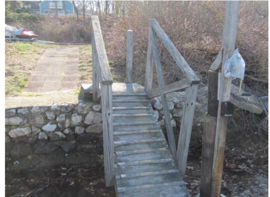
Deteriorated wood platform and ramp
