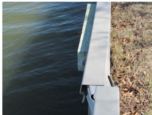
Aluminum bulkhead reinforced with wood rail
