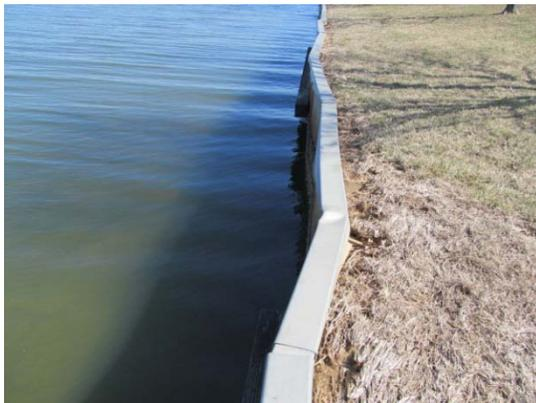
Aluminum bulkhead displaced
